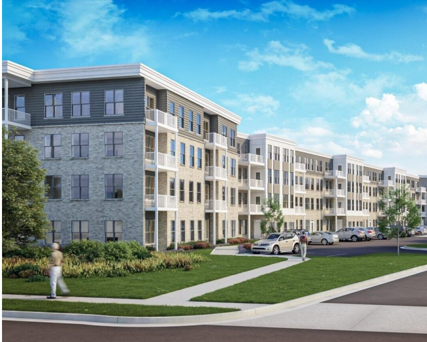
Apartments under construction in Rock Hill, representing a type of housing that employers suggest is undersupplied in many parts of the region.
